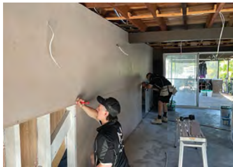
Workers repairing the Kriesch's home.
