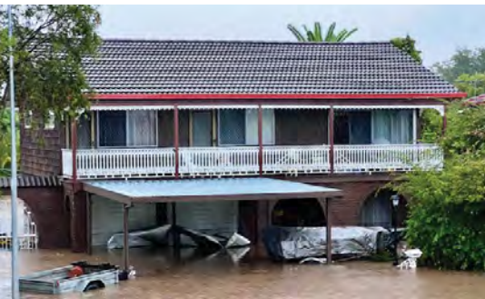
Floodwaters inundated the home of Elizabeth and Kevin Kriesch.
