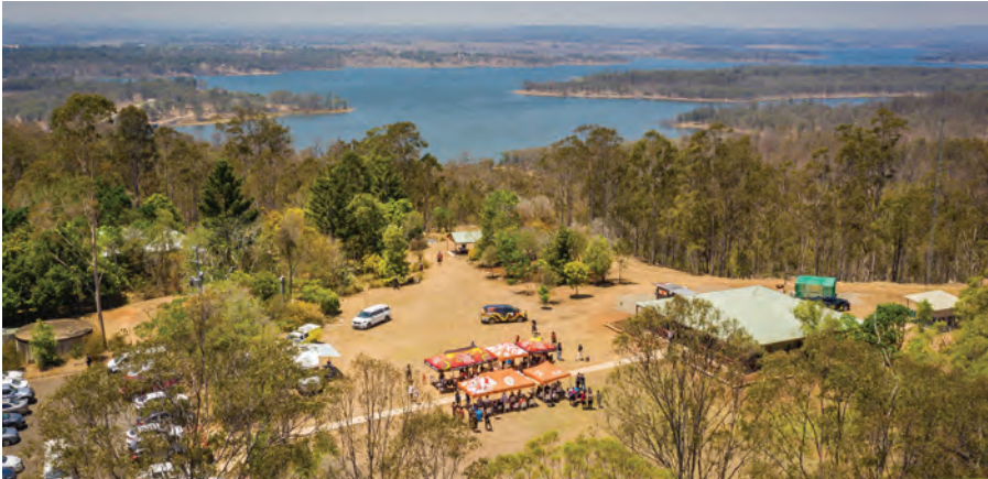
An aerial view of Bert Button Lookout with Bjelke-Petersen Dam in the background.
